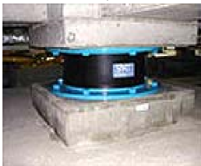
Figure 3. Base Isolation Device
